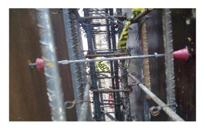
Technical Name: Steel formwork spreaders Commercial Name: Snap Tie
